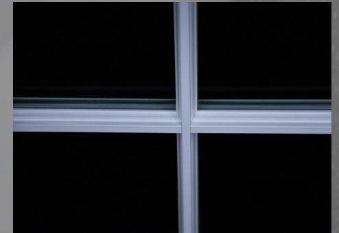
Exterior and interior muntin bars are treated to match sash, either with exterior paint, or interior lamination.
