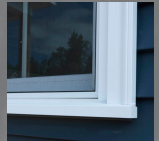
Historic accuracy is maintained with the joinery of our 5/4 x 3 1/2" Flat (left) Staff Bead Brickmould (above), or 4 1/2" Banded (below) with our Historic Sill Nose.
