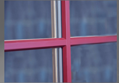
Exterior and interior muntin bars are treated to match sash, either with exterior paint, or interior lamination.
