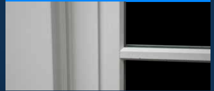
Classic Blind Stop Face Mounted Casing
